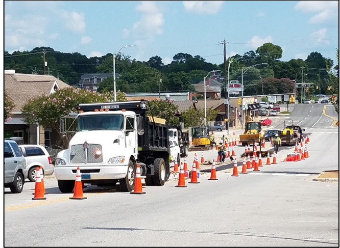
Sewer Main Replacement Project on College Street
