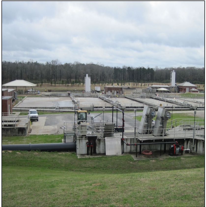
H.C. Morgan Water Pollution Control Facility
