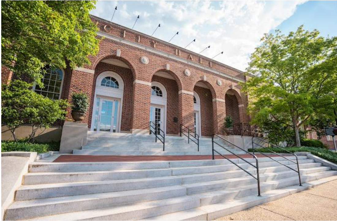
City of Auburn City Hall
