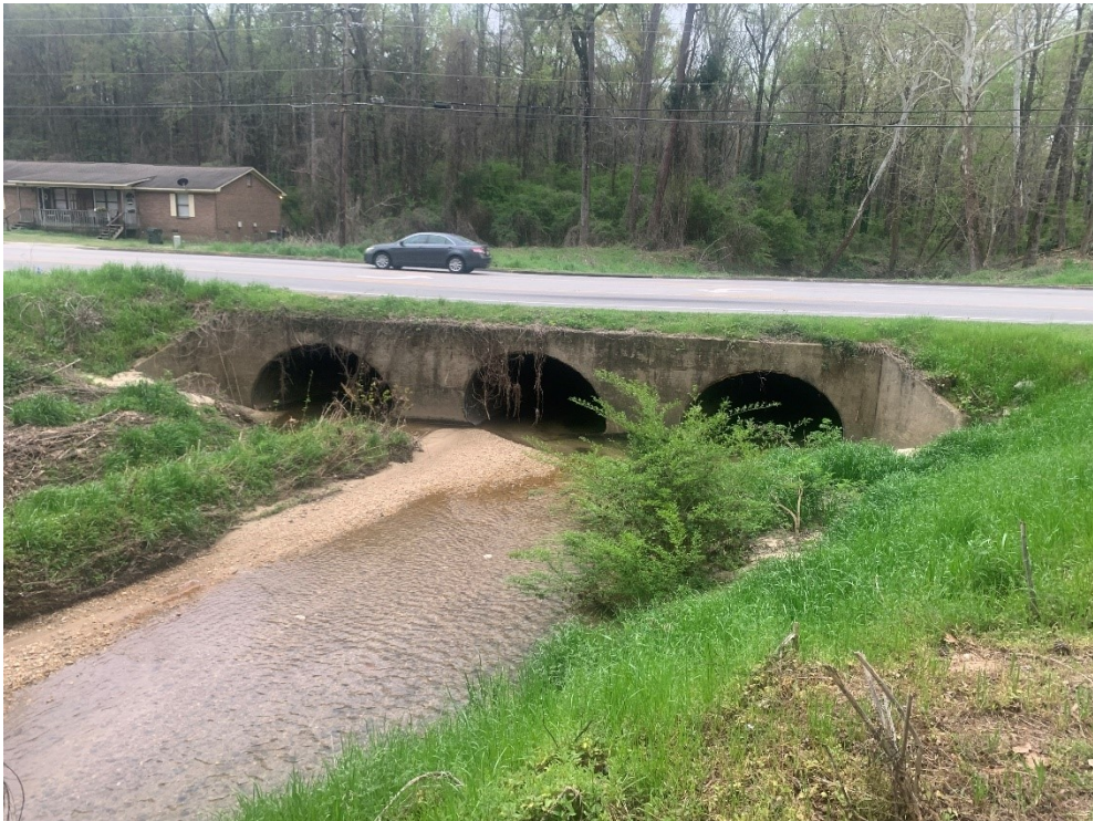
Figure 2: North Side of Existing Culvert Facing South
