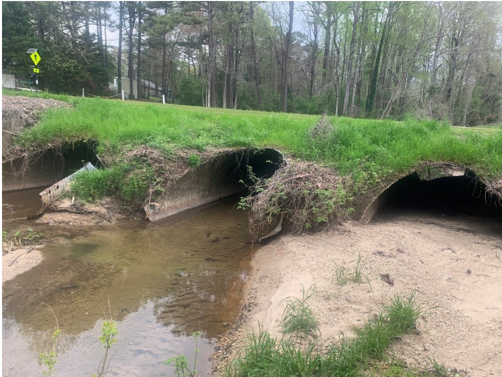
Figure 3: South Side of Existing Culvert Facing North
