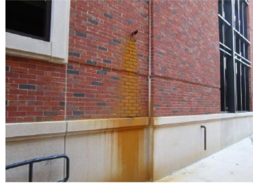
Photo 15 – Staining present on south side of garage exterior under pipe extending through wall from generator room
