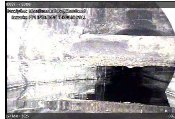
Figure 2.4 - Grade 5 Pipe (B0099-B0098: pipe obstructed by utility crossing)
