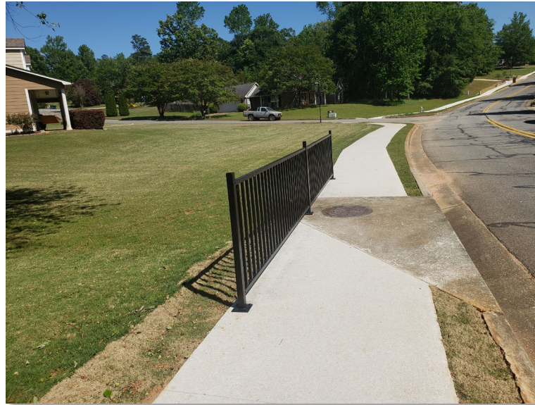
Drainage and Handrail Improvements
