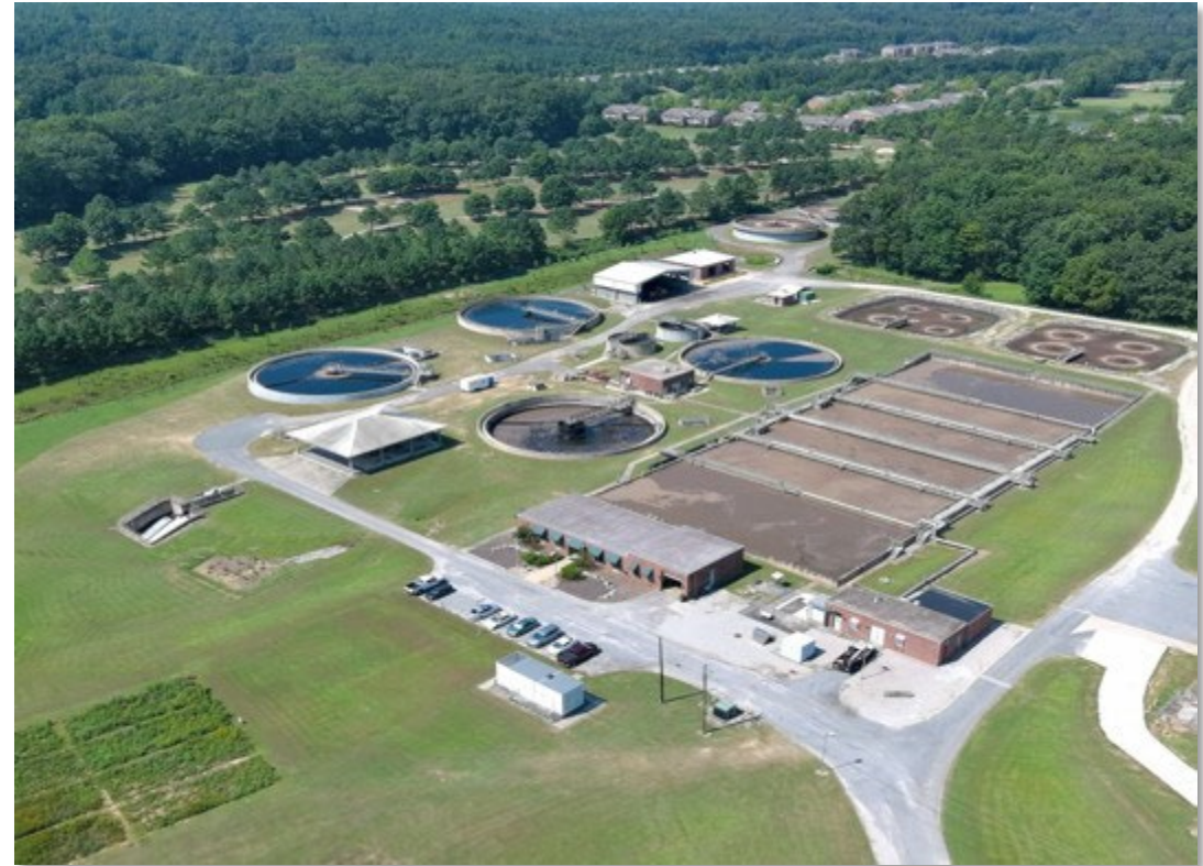
H.C. Morgan Water Pollution Control Facility (August 2024)
