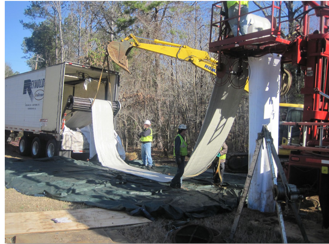
Sewer CIPP Lining Project
