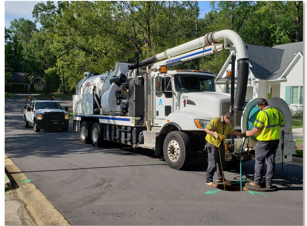
Sewer Line Cleaning
