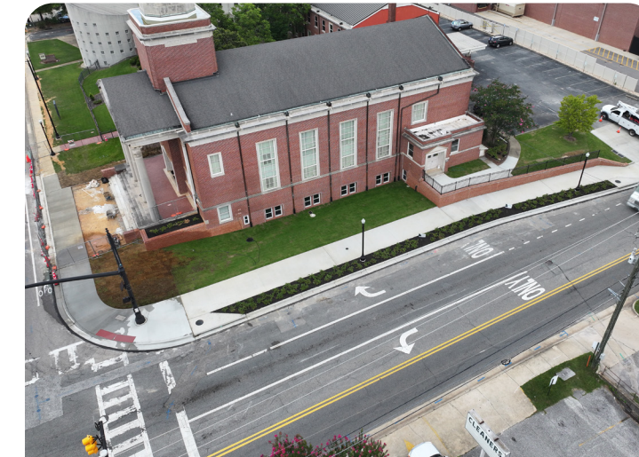
Gay Street streetscape project
