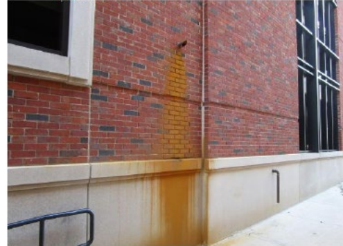
Photo 15 – Staining present on south side of garage exterior under pipe extending through wall from generator room
