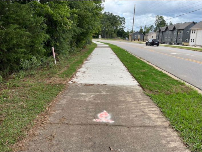
>9,000 Linear Feet of Sidewalk Patches
