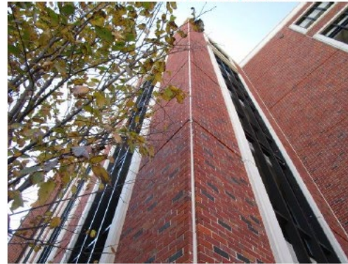
Photo 16 – Exterior joint sealants generally appear to be in good condition
