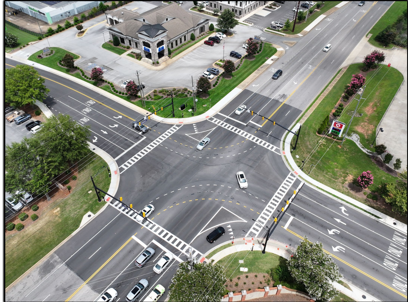
North Dean Road at East University Drive Intersection Improvement Project
