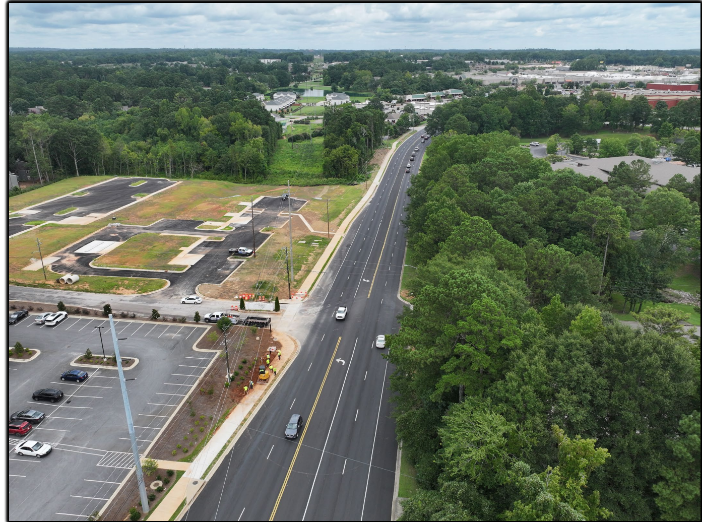
East University Drive at Stoker Intersection Improvement Project
