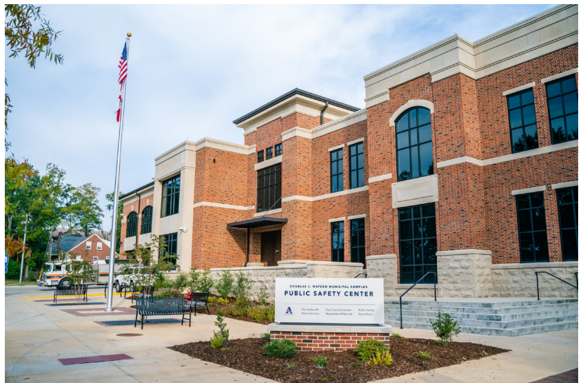
Public Safety Complex
