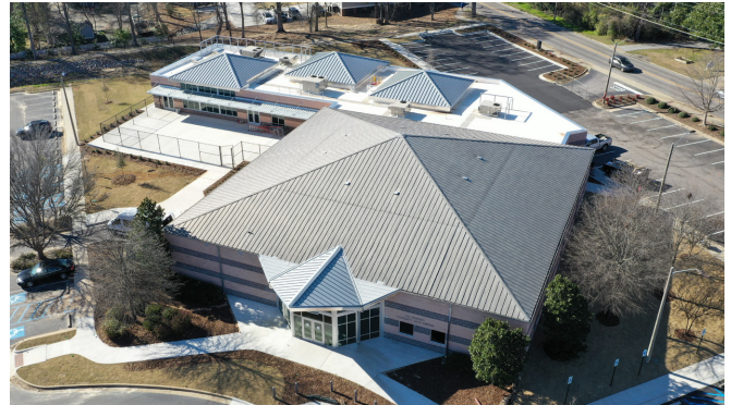
The 10,000-square-foot facility was renovated and an 8,000-square foot addition was constructed.
