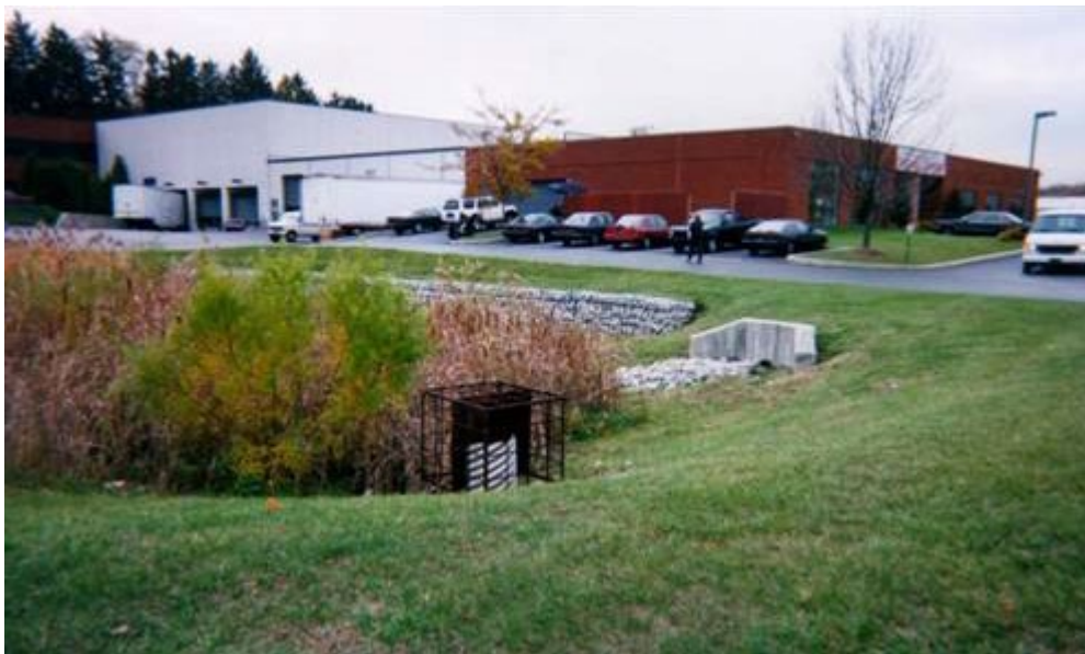
FIGURE 4-29 Dry Extended Detention Basin with Shallow Marsh
