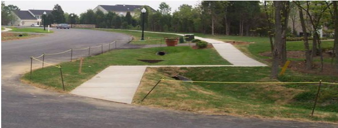
FIGURE 4-9 Recently Constructed Grassed Swale in Residential Area, Pembroke Woods Subdivision in Emmittsburg, MD (Courtesy of Mike Clar, Ecosite, Inc., Columbia, MD)
