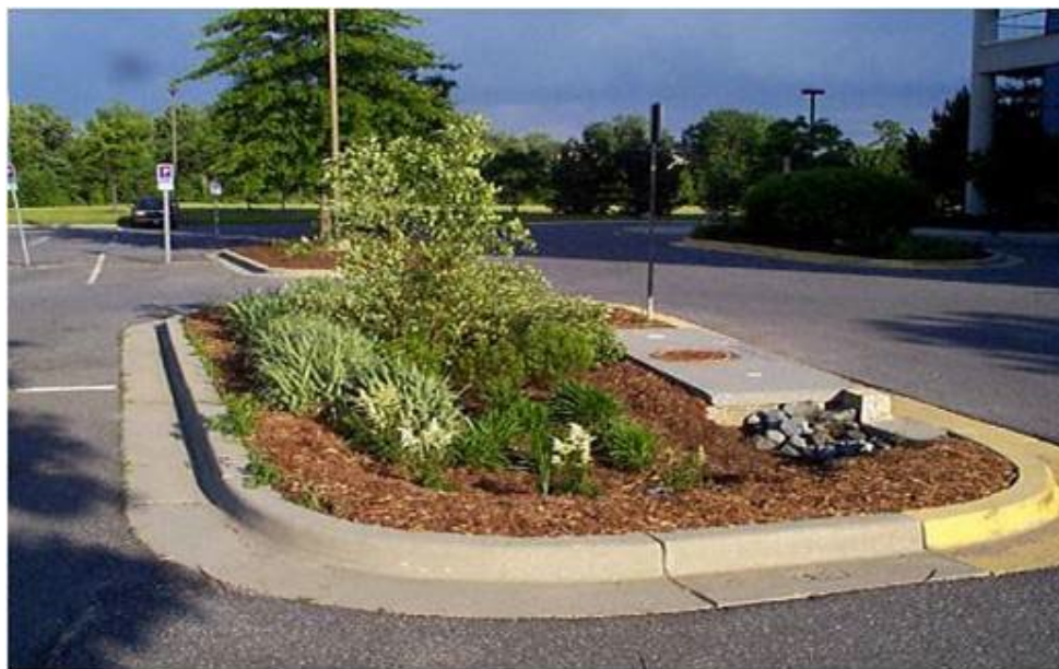
FIGURE 4-3 Bioretention in Parking Lot Island
