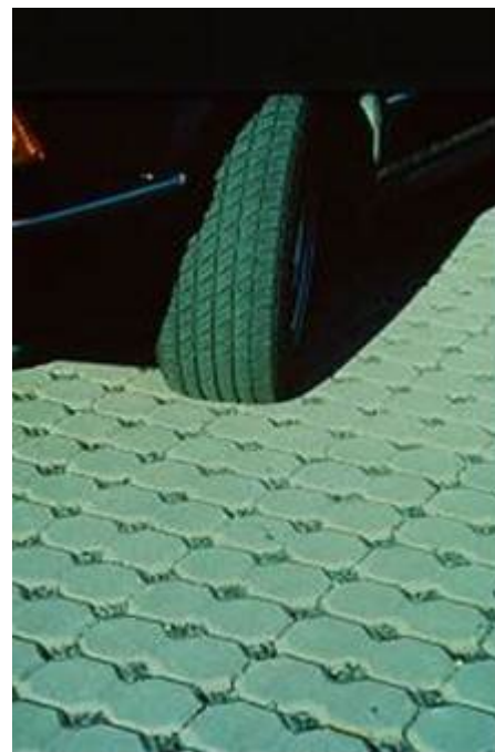
FIGURE 4-17 Parking Lot with Interlocking Concrete Grid Installation (Courtesy of the Interlocking Concrete Pavement Institute)
