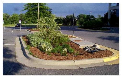
FIGURE 4-3 Bioretention in Parking Lot Island
