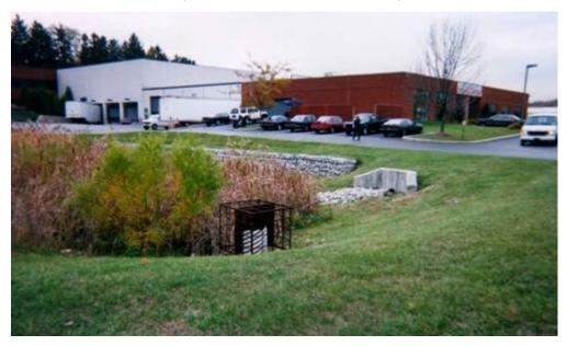
FIGURE 4-29 Dry Extended Detention Basin with Shallow Marsh
