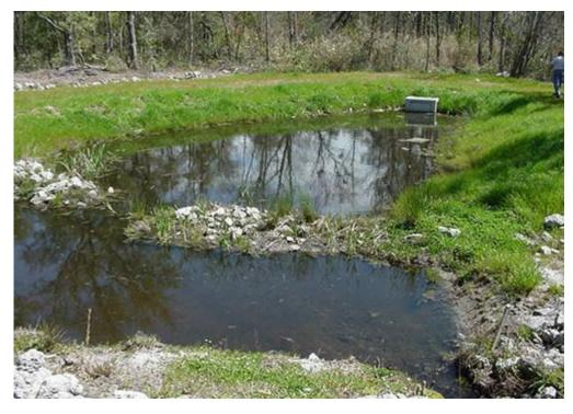
FIGURE 4-8 Permanent Pool of Water in Wet Detention Basin
