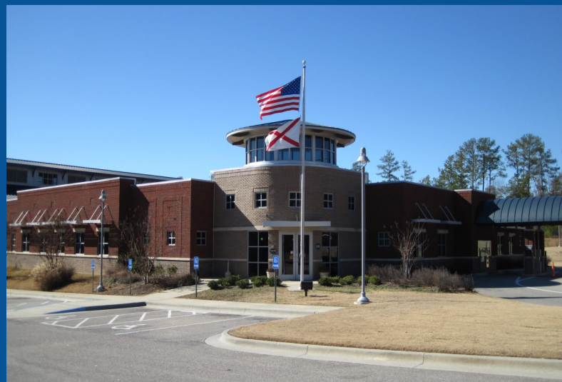
Below: The Bailey-Alexander Water and Sewer Complex houses field operations, administration, and billing services.
