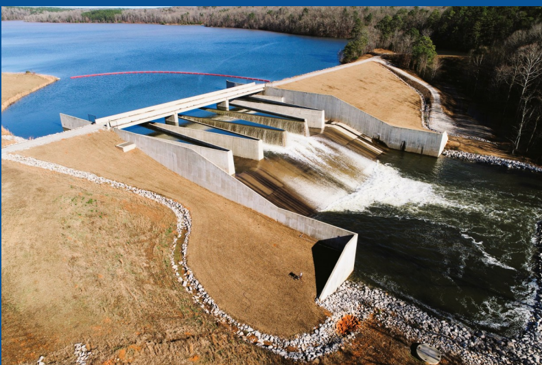
Above: Completed in 2017, the new spillway added 50 million gallons of capacity to Auburn's primary water source, Lake Ogletree.
