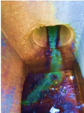
**Illicit Cross Connection** - A sanitary sewer line that is either directly or indirectly discharging sanitary sewer to our storm sewer system.
