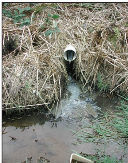
Figure 2: Direct Discharge from a Straight Pipe
