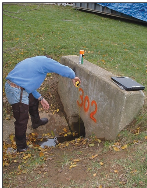
Figure 10: Measuring an outfall as part of the ORI
