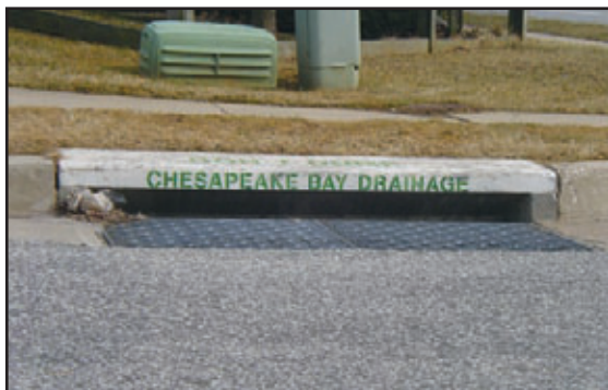
Figure 14: Storm drain stenciling may help reduce illicit discharges.
